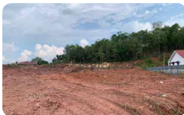
Taman Paloh Phase 2 - site clearance
