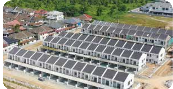
Taman Perdana Putera Phase 1 - in progress
